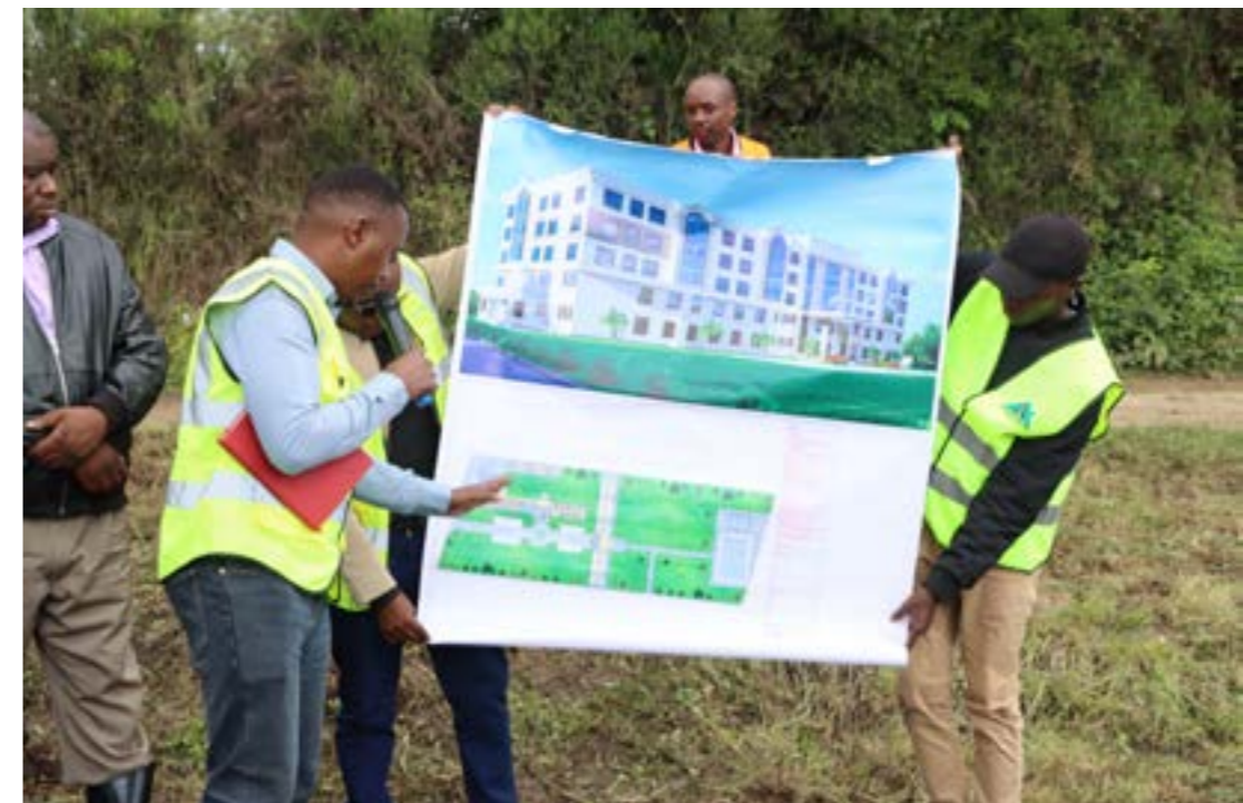
Members of the technical team presenting the architectural design of the Sabbatical Centre
